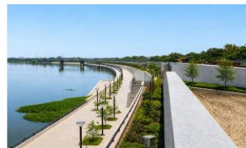
Foundation and Specialist Engineering ₹1,296 Cr | 4%
