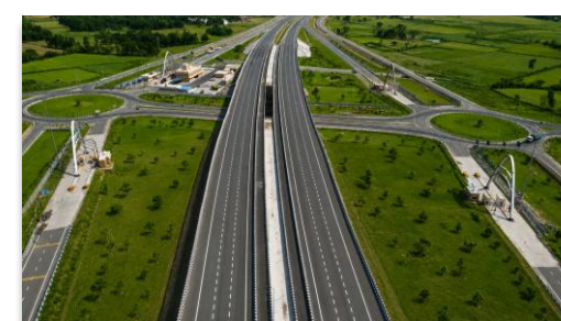
Ganga Expressway, Uttar Pradesh
