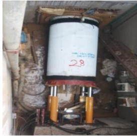
Micro Tunnel Boring Machine (5 Units)
