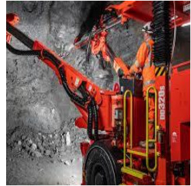
Twin Boom Jumbo Drill (8 Units)
