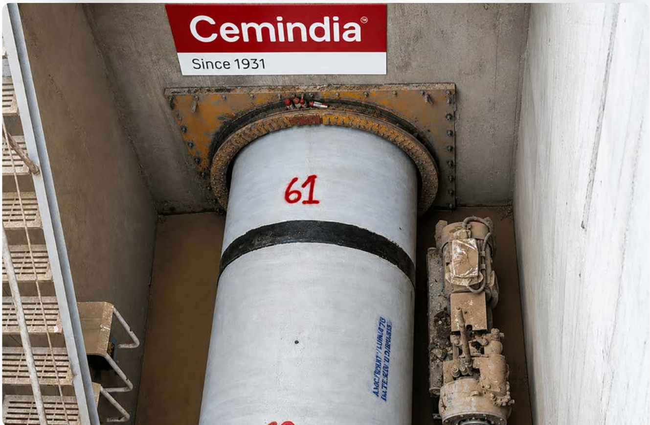
▲ Ahmedabad Micro-tunnelling Project in Gujarat
