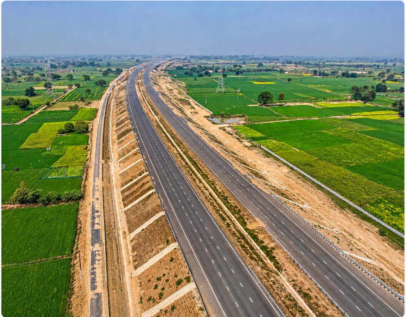
▲ Ganga Expressway Road Project in Uttar Pradesh
