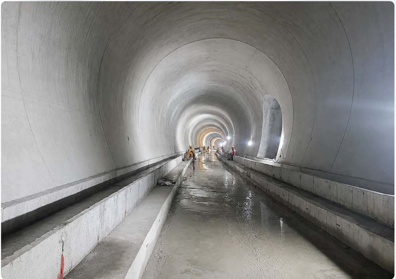
▲ Sivok Rangpo Railway Tunnel in West Bengal and Sikkim
