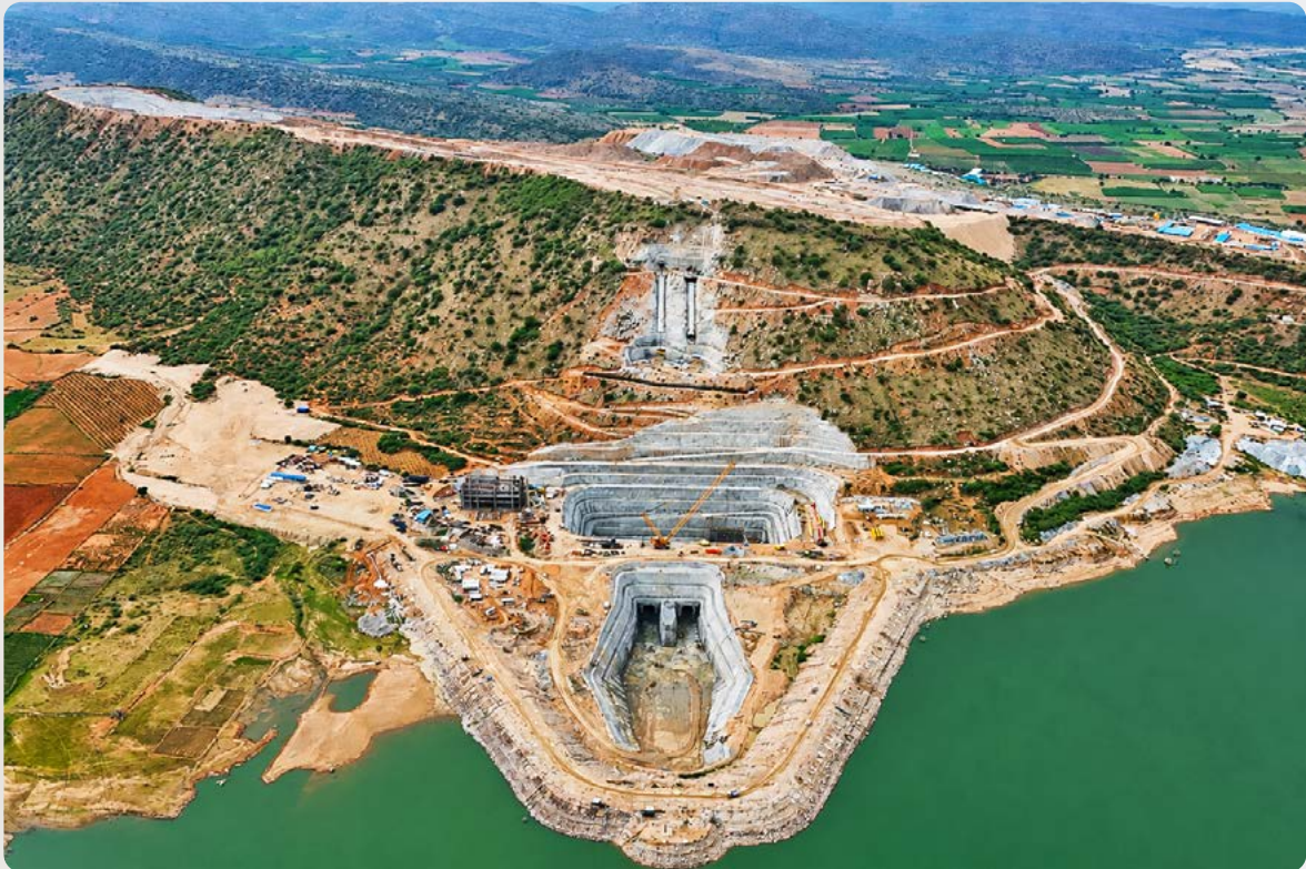
▲ Chitravathi Pumped Storage Project in Andhra Pradesh
