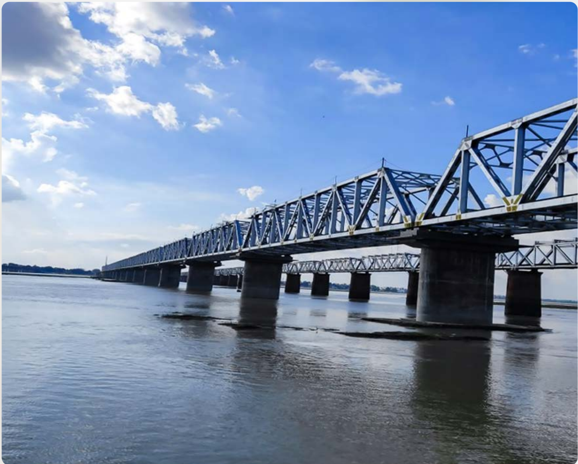
▲ Steel Bridge over River Ganga in Uttar Pradesh
