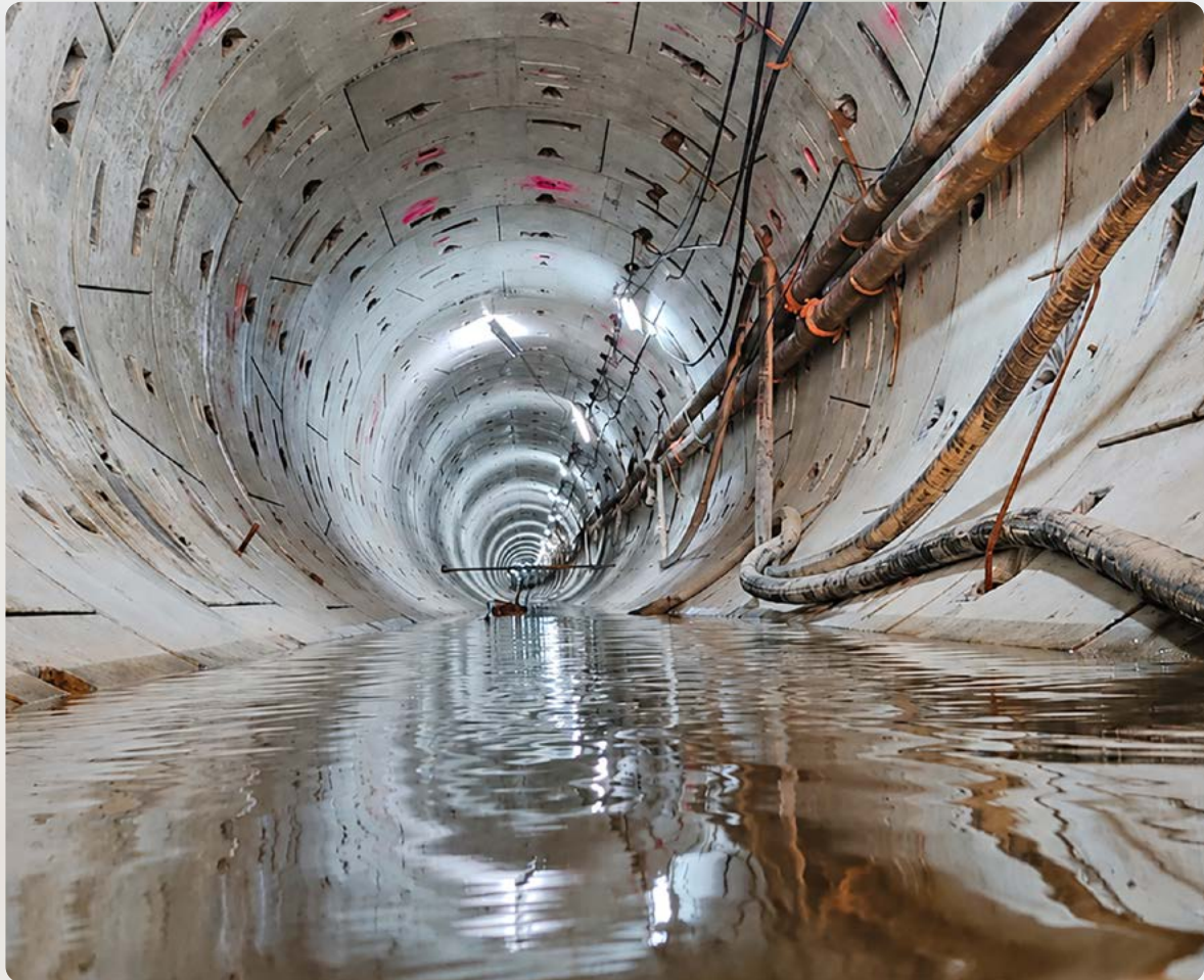
▲ MCGM Micro-tunnelling Project in Maharashtra
