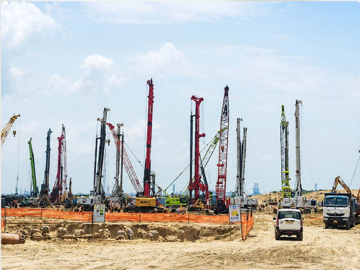
▲ Piling Work at JSW Utkal in Odisha
