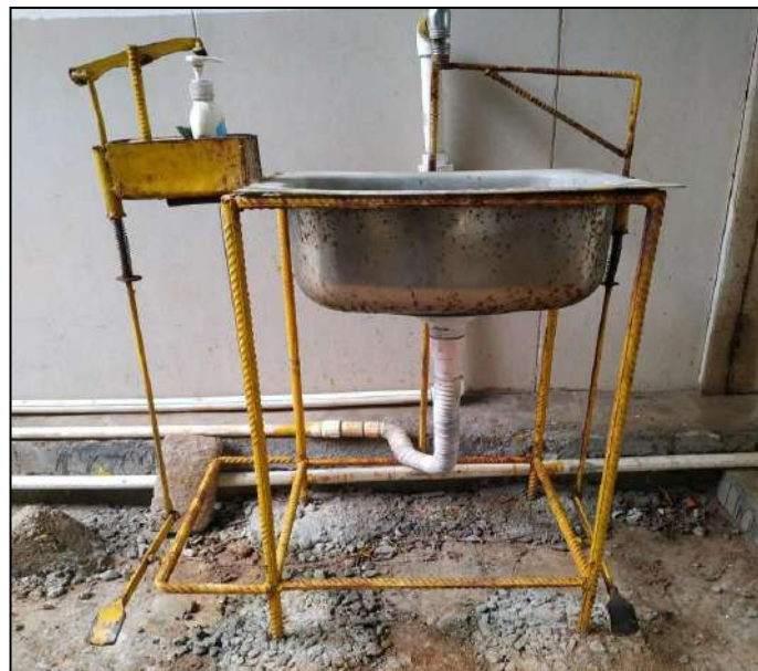
Hands Free Sanitizer & washing facility at Airport AAI - Trichy Project (EA-045718)
