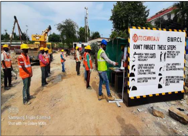
Following good Hygienic practices at R1A-BMRCL Piling Project (A1617BWD3)
