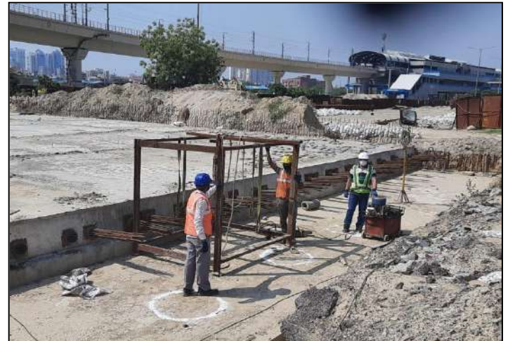
Maintaining Social Distancing while working at Noida Underpass -(CW-047619)
