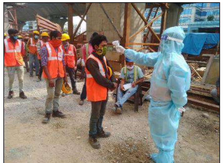
Regular Thermal Temperature Screening at BMRCL R5-P2 (A1917BW-D2) Project Site
