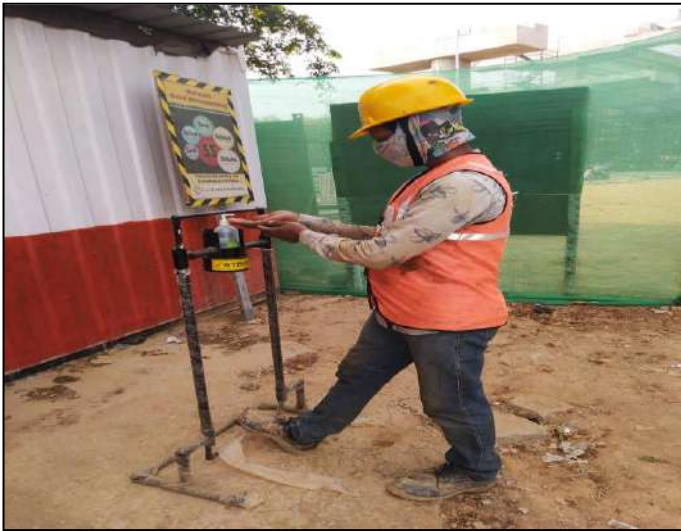
Provision of Hands free Sanitizer at Site A1717BW-D2 (BMRL R1B) Project
