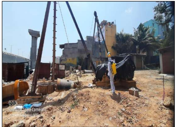
Sanitization of Work place at R1B-BMRCL Project (A1717BWD3)
