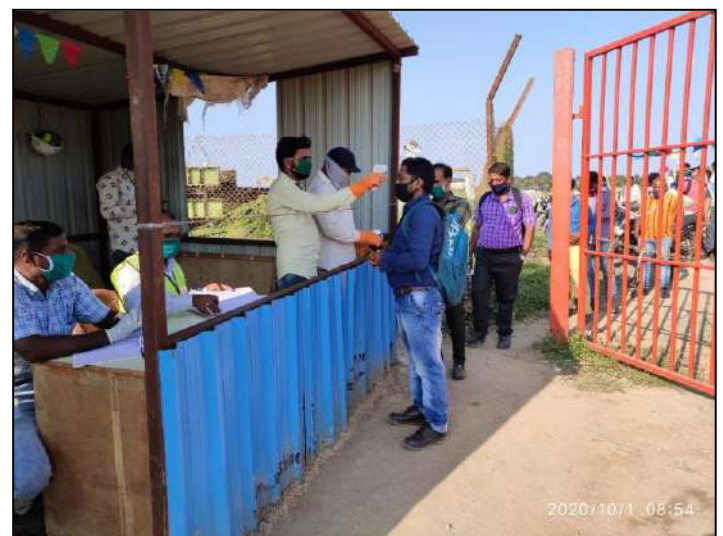
Temperature screening at the entrance of Chhara Port Project Site, Gujarat (47119 DM)
