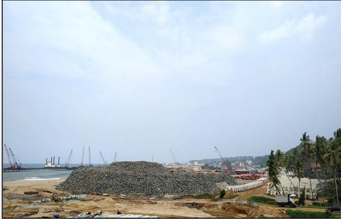
Vizhinjam Break Water Project
