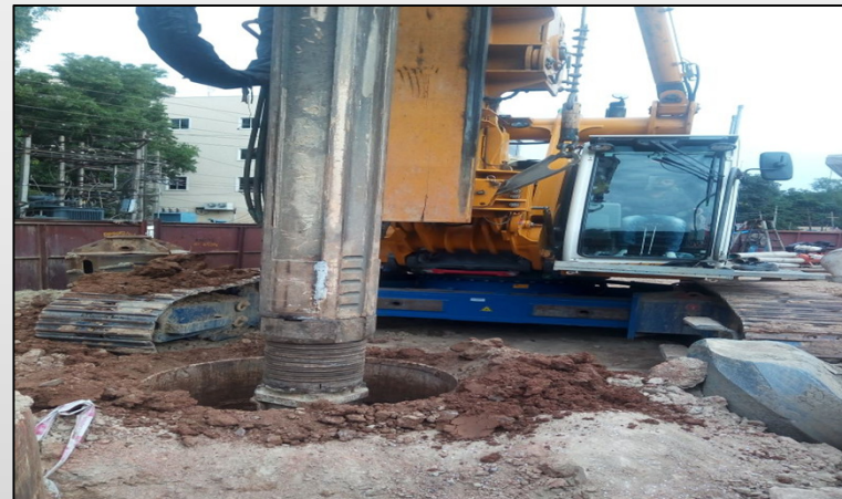
Piling Work at Bangalore Metro
