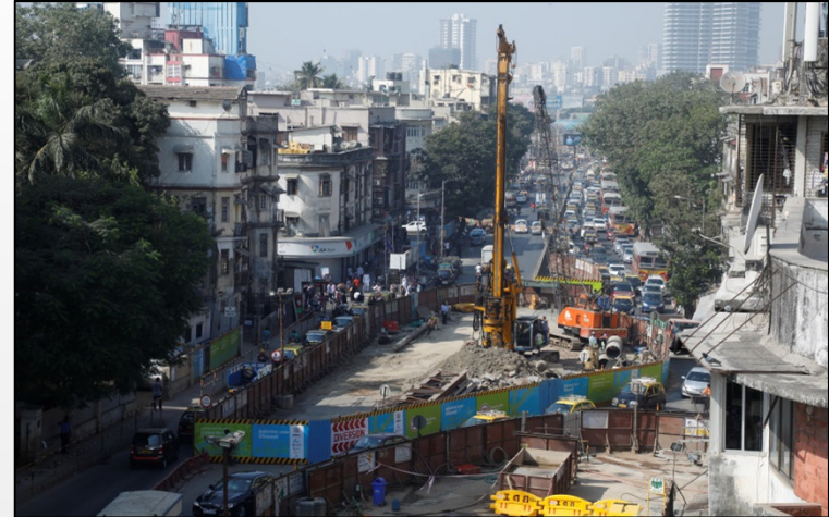
Piling Work at Mumbai Metro
