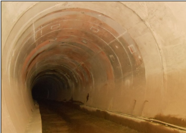
Tunnel for Indian Railways
